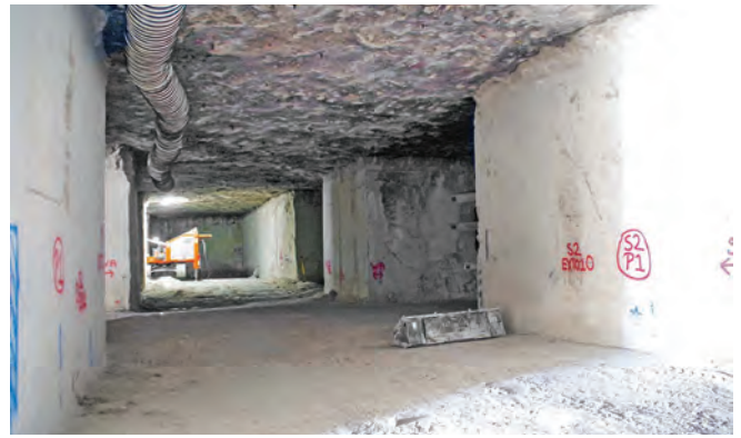
Cutting machine is seen in the cross alley
